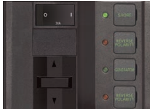
Circuit Breaker Source Selection
