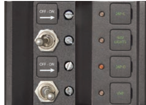
COTS Circuit Breaker
